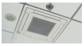
The Daikin *VISTA* Ceiling Cassette fits within a 2'x 2' ceiling grid and can be installed in close proximity to other building accessories.
