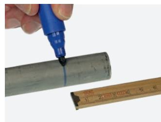
The required insertion depth (table in step 7 of installation guidelines) must be marked on the pipe in order to guarantee a safe and proper joint. The fittings with pipe ends already have a pre-marked insertion depth, thereby rendering any
