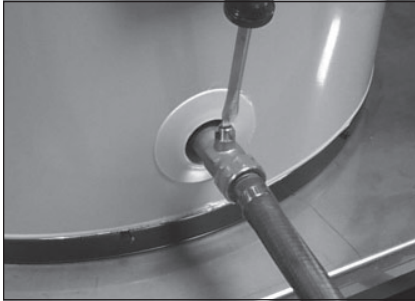
Figure 10 - Draining the old water heater.
