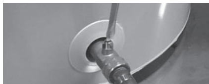
Figure 28 - Drain Valve
