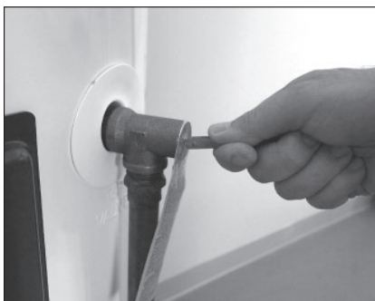
Figure 40 - T&P Relief Valve
