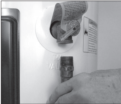
Figure 11 - Removing the T&P Relief Valve discharge pipe.
