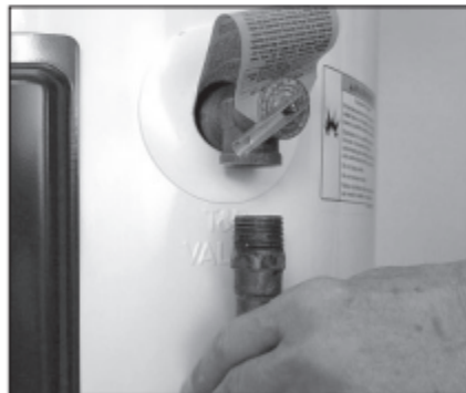
Figure 11 - Removing the T&P Relief Valve discharge pipe.
