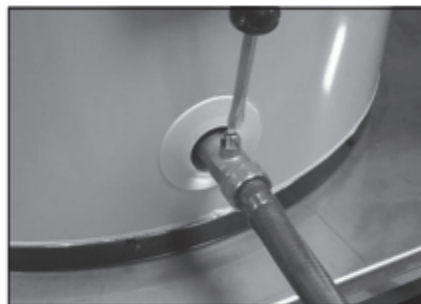
Figure 10 - Draining the old water heater.
