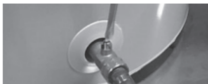
Figure 28 - Drain Valve
