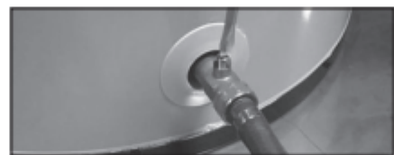
Figure 37 - Drain Valve
