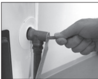
Figure 40 - T&P Relief Valve
