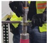
10. Verify the location marking on the outlet reducer and match the outlet location for the remaining head installations.
