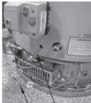
PILOT FEEDLINE — MAIN BURNER FLEXIBLE FEEDLINE
