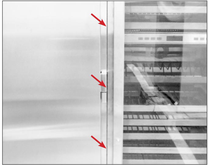
FIG. 16. Verify the gap(s) between cabinets is (are) even throughout.
