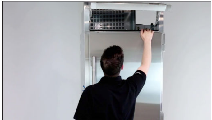
FIG. 3. Be sure to inspect behind the rainshield.
