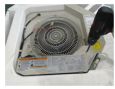
Fig. 14 —Open Control Box Cover
