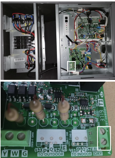
Fig. 29 — Connect the auxiliary heat wire
