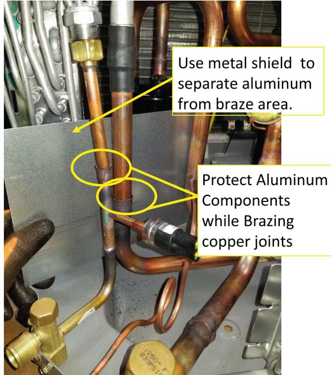
**Fig. 32 – Use Braze Shield to Protect Aluminum**
