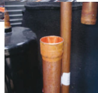
Fig. 12 – Bell Suction Tube
