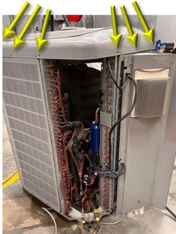
Fig. 3 – Top Cover Screw Locations
