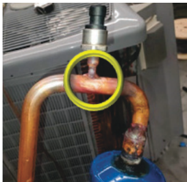
Fig. 4 – Braze Pressure Transducer
