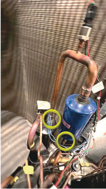
Fig. 13 – Braze Joint Locations
