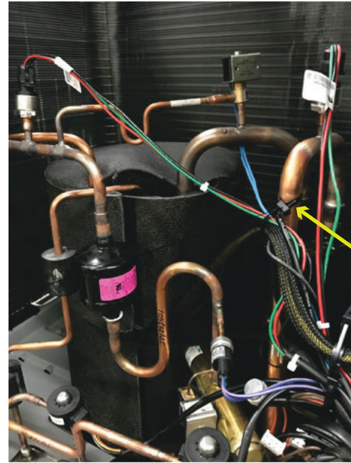
Fig. 6 – Cut wire Tie on suction Tube
