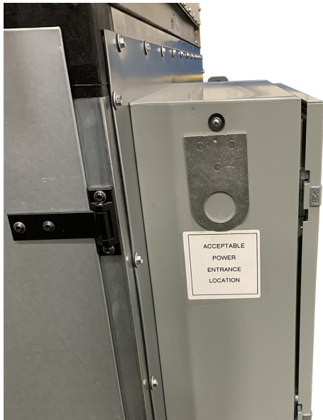
Fig. 182 — Acceptable Power Entrance Location
