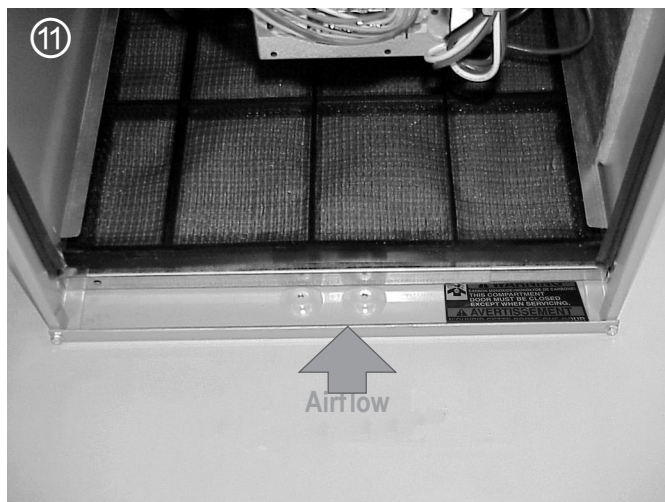
BOTTOM FILTER RACK INSTALLATION
