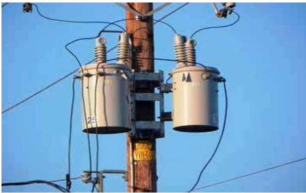
Open Delta (Wire Connection)
