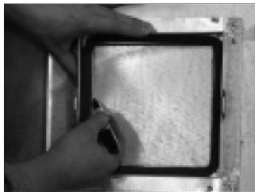
2. Using a hand held plasma cutter or by conventional methods, cut the hole for the frame.
