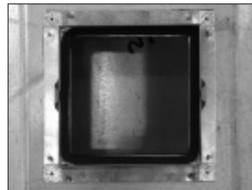
5. Using zip screws, permanently attach the frame to the ductwork. Doors 16" and smaller require one screw at each corner and one at center on each side. Doors 18" to 24" require one screw at each corner with two screws evenly spaced on each side of the frame.
