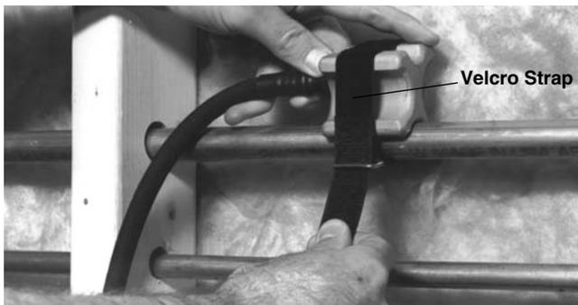
Figure 5 – Applying Freeze Head with Velcro Strap
