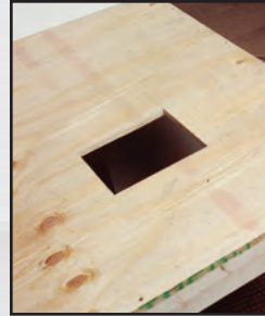
Cut the hole.
