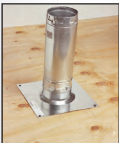
Continue adding pipe sections - supports up to 90 lbs.
