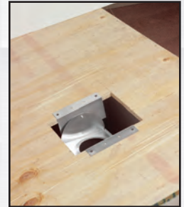
Mount SureGrip support plate.
