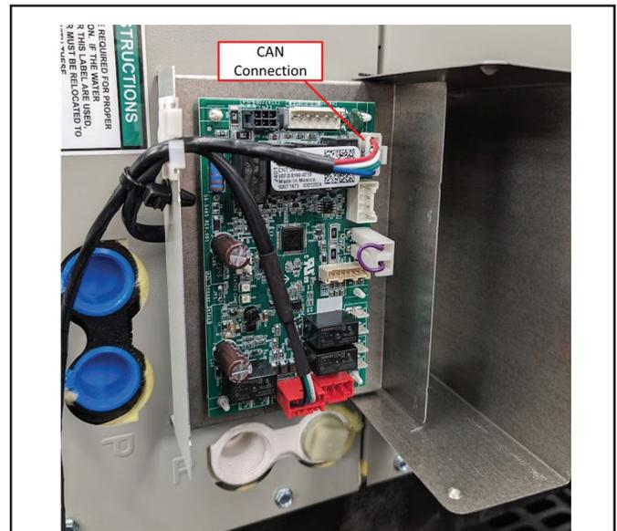
Figure 20: Comm/Link harness connection to MCB
