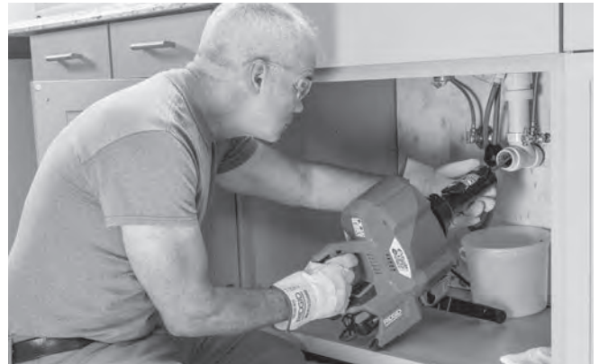
Figure 13 – Feeding Cable With AUTOFEED Unit
