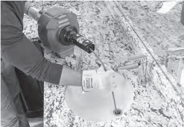
Figure 14 – Manually Feeding Cable
