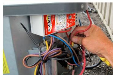
13. Remove the loose wire (from Step 7) from the active input of the contactor and attach the stripped end of the Active wire in its place.
