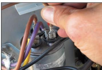
7. Identify the cable connecting the contactor and the Run Cap. Remove this connection to the Run Cap. Attach the flagged end of the brown wire to the same terminal of the Run Cap<sup>#1</sup>.
