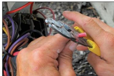
4. Strip the compressor Run wire at least 1/2 in\*. Crimp appropriate size Ferrule (supplied) onto it.
