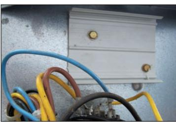
2. Secure the mounting bracket for the NuStart inside the control
