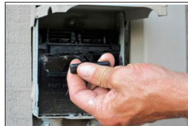
1. Turn off all power to the HVAC unit at the circuit breaker.
