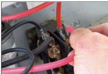
3. Remove the compressor Run wire from the contactor or Run Capacitor terminal, as applicable.
