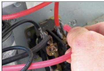
3. Remove the compressor Run wire from the contactor or Run Capacitor terminal, as applicable.
