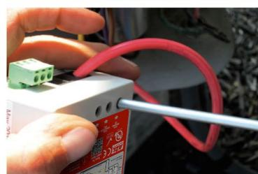
5. Attach the compressor Run wire to the NuStart Run Winding terminal.
