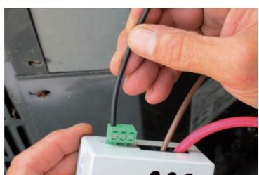
8. Attach the black wire (supplied) to Compressor Common on the NuStart green terminal connector.
