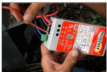
12. Attach the red wire (supplied) to the Active Terminal on the NuStart.
