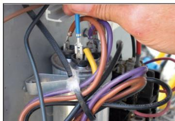
11. Attach the flagged end of the blue wire to the other terminal<sup>#2</sup> of the Run Capacitor. Ensure that this terminal on the capacitor also joins to the Start Winding of the compressor.
