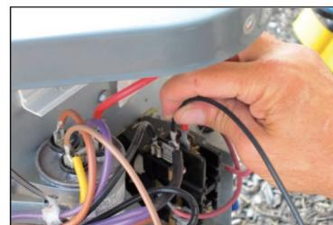
9. Attach the flagged end of the black wire to the Compressor Common on the "T" side of the contactor.
