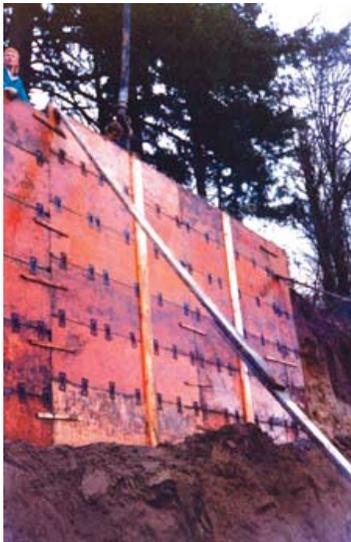
The key to the RAP-I-FORM® system is a spreader type clip that fits over the top of, and under the bottom of, the forming plywood. On the job, form clips are laid out on a pre-poured footing and spaced approximately two feet apart. HDO plywood, cut into 2'x8' sheets, is then set into the form clip. Top clips are then applied to hold the top of the form in place, and the foundation wall is poured.
