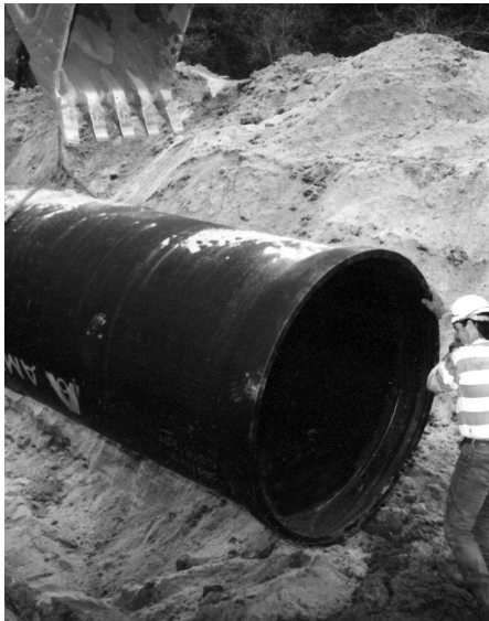
64" AMERICAN Fastite Joint pipe being installed in a wastewater application.
