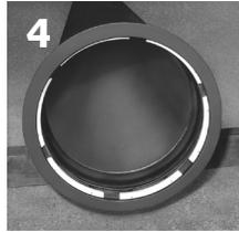
**(1). Important: A Fastite gasket must also be used, because the rubber-backed flex-ring does not perform any sealing function. 2) Placement of the flex-ring in socket and joint lubrication**
