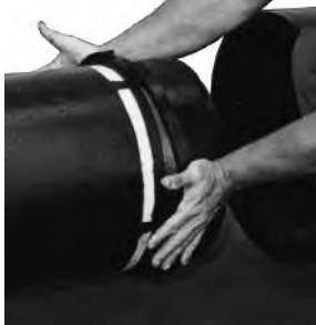
FIELD ASSEMBLY OF FLEX-RING
