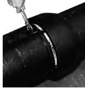
DISASSEMBLY OF 4"-12" FLEX-RING
