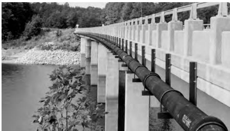
This bridge crossing illustrates design/construction advantages, including the deflection capabilities of AMERICAN Flex-Ring Joint Pipe.
