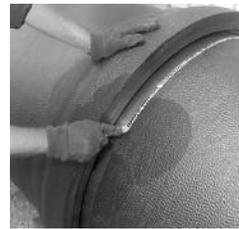
E) After all shims are inserted, place a reference mark on the spigot even with the exposed end of the shims. Pull, jack, or deflect the spigot out from the socket.
