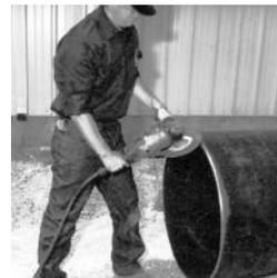
A portable grinder should be used to make a bevel 3/8" to 5/8" long at an angle of 30-40° with the axis of the pipe. All sharp corners or rough edges that might damage or dislodge the Fastite gasket
