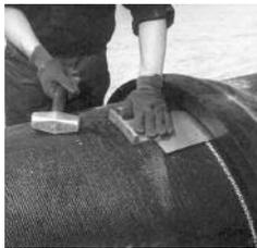
C) Carefully drive a disassembly shim between the gripping teeth of the segments and the spigot with a hammer. Lifting or offsetting of the spigot relative to the
