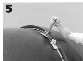
\*Note: The lok-ring is normally shipped in position on the pipe plain end behind the welded-on retainer ring. See page 9-25 if field assembly of lok-ring is required.
