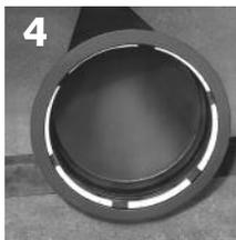
segment fits reasonably flush against the wedging surface of the socket, and no rubber bulges or twists remain (Photo 4).
