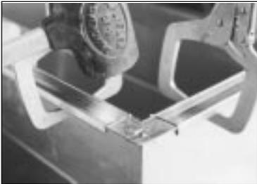
7. Use a mallet to seat the frame onto the duct. *Establish metal to metal contact along length of the angle.*
