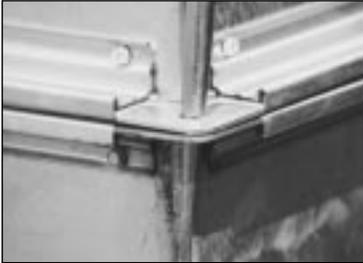
15. Carefully align mating frames before they touch. Ductmate 440 adheres on contact. A drift pin can be used to correct any misalignment.
