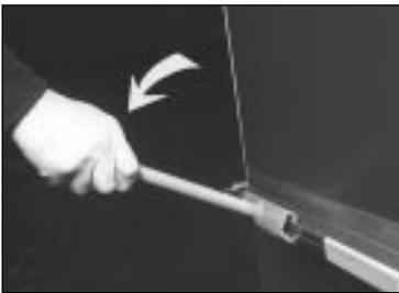
17. WDCI cleat can be snapped-on with the Snapper 1 Tool or with the Snapper II where space is restricted.
