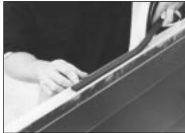
2. Start applying Ductmate Neoprene gasket about halfway between corners. Position gasket in center of WDCI angle as in photo.
