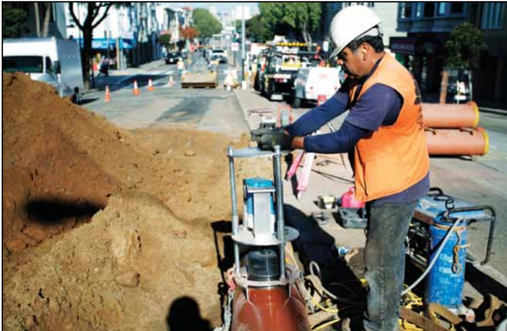
Joints' specially designed coring machine is designed specially for sewer and drain pipe drilling above or below ground.
