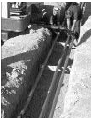
Fig. 6-1. During layout, bonding and inspection, support the piping on 2x4 "batter boards" to keep the joints clean and to keep bedding out of the pipe.
