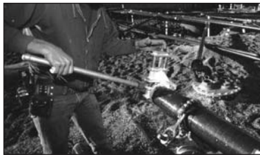
Fig. 5-3. Dualoy 3000/LCX can be tapered using the Ameron Taper Maker. The ratchet handle makes the Taper Maker convenient to use in confined spaces when repairing existing lines.
