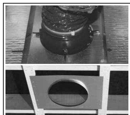
Use optional DCF Flange for added strength in T-bar applications or RCF16 and RCF24 for new work at the rough in stage.
