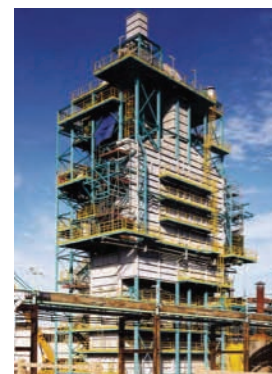
Ethylene Cracker Unit
