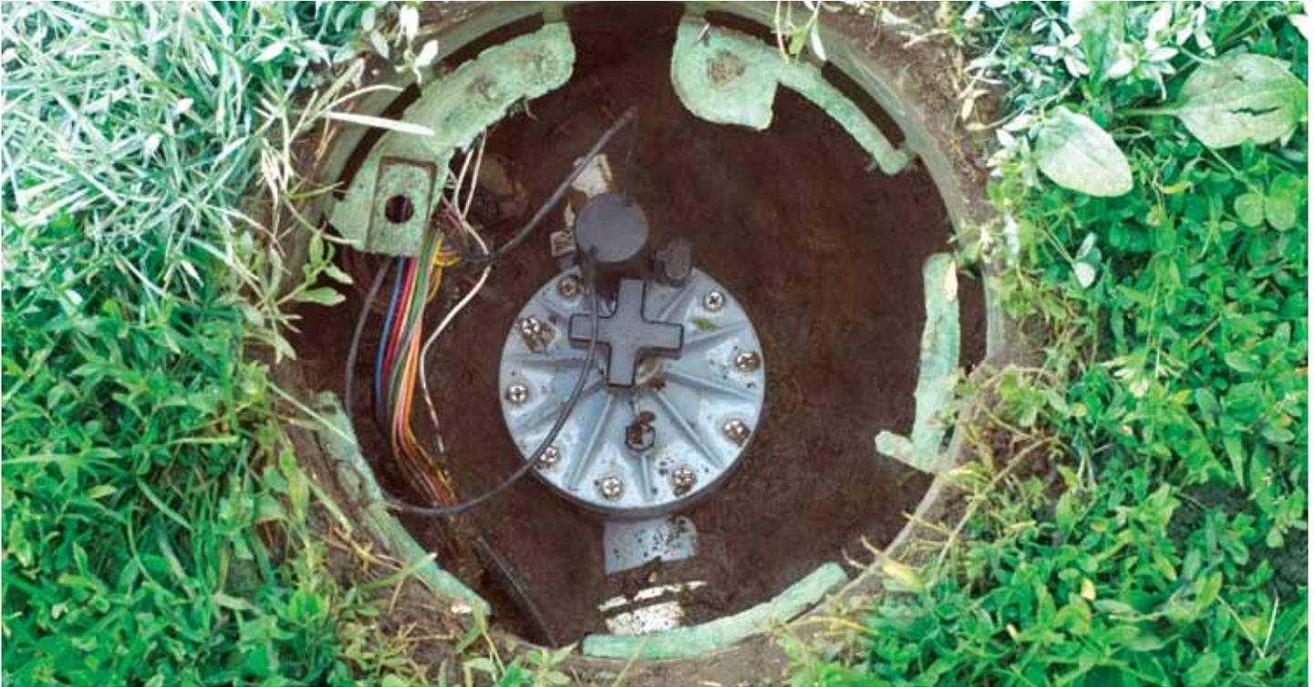
The Irritrol® 200B Series globe/angle valves have built their popularity on a proven record of reliability and a reputation for offering valuable features at an affordable price. The 200B Series provides manual internal and external bleed, heavy-duty, UV-resistant PVC construction, stainless steel hardware, a double-beaded diaphragm and a captive solenoid plunger.
