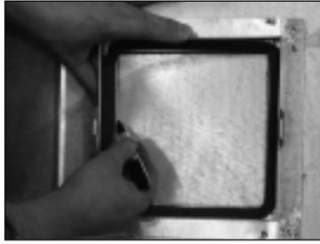
2. Using a hand held plasma cutter or by conventional methods, cut the hole for the frame.
