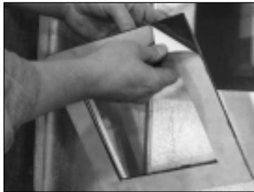
4. Open the door and place the frame over the hole you cut in step 2.
