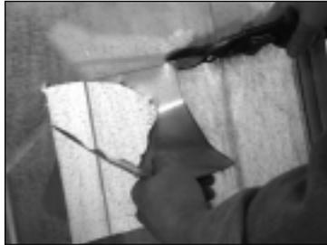
3. Remove the cover from the adhesive backed gasket tape.
