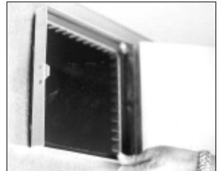
4. Bend over all of the dovetails on the frame with a hammer to ensure a tight fit.
