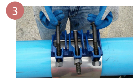
3 Tuck the gasket flap in place, close the bolt lug, engage the centermost bolt(s) and finger tighten. NOTE: using the palm of your hand, squeeze the end of the clamp fingers and the top of the stud lug to bring stud bolt and fingers parallel.
