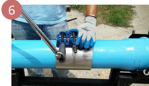
Allow the gasket to fully compress, and recheck the bolt tightness. It is important to re-torque Tapped Repair clamps when used as a "hot tap" saddle after the tap has been made. Torque the bolts as evenly as possible:
