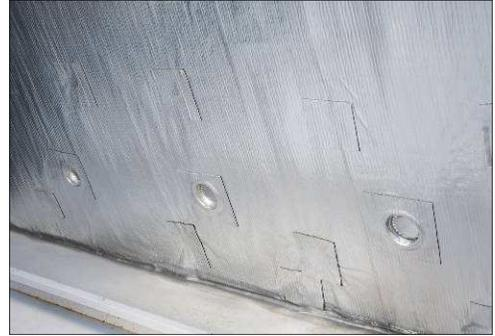
On ducts over 24" (60 cm) in width, pin bottom on 12" (30 cm) centers. Cover pins with a 3" (8 cm) square minimum of FlexClad.
