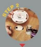
Put toilet flange onto drain and make solvent weld connection.
