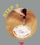
Secure toilet flange to floor with fasteners.
