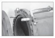
8. TIGHTEN DRAW BOLTS: After the four assembly bolts are inserted into the lap-joint bolt holes, torque the draw bolts to approximately 150 ft-lbs/203 N•m. NOTE: It is normal to have a small amount of shift as these bolts are being torqued.
