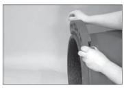
**ADD FIRST SEGMENT: Place** the first segment onto the pipe, making sure that the key engages in the groove properly. NOTE: On vertical pipe, the segments must be held in place until all segments are fastened together. For horizontal pipe, the segments can be balanced on top of the pipe, as shown above.
