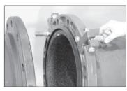
7. INSERT STANDARD FULL-SHANK DIAMETER ASSEMBLY BOLTS AT LAP JOINTS: Insert a standard, full-shank diameter assembly bolt into each of the four lap joint holes. NOTE: It may be necessary to tighten the draw bolts to line up the lap joint bolt holes for insertion of the bolts.
