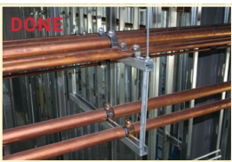
Level, tighten lock nut
