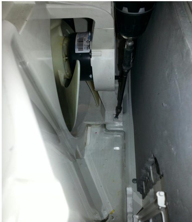
**Figure 410 (Remove Gussets and Fan Shroud)**
