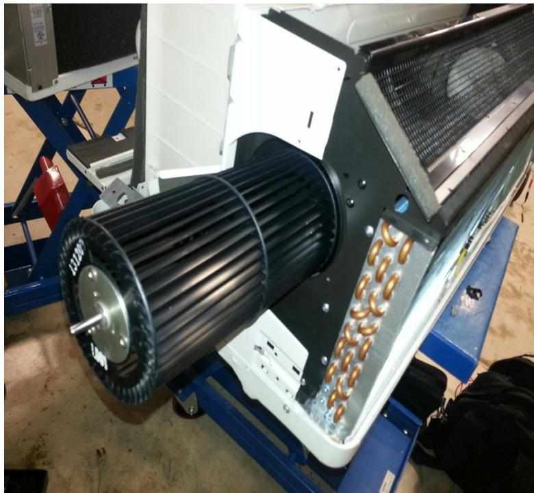
Figure 405 (Removal of Indoor Fan Blower Assembly)
