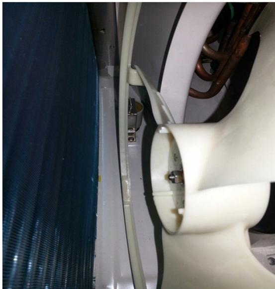
**Figure 411 (Loosen Fan Shroud and Bellows Drain Valve Located inside Shroud)**
