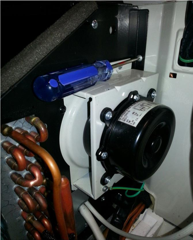
Figure 406 (Removal of Indoor Fan Housing Assembly)
