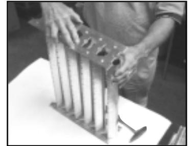
4. Insert vane and rail assembly into the ductwork and secure using standard self-drilling screws. *Secure rail to ductwork per SMACNA standards.*
