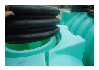
4. Drill four 1" holes at approximately 90 degrees from each other in bottom rib as shown.
