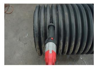
2. Pipe cut. Deburr edges with file.
