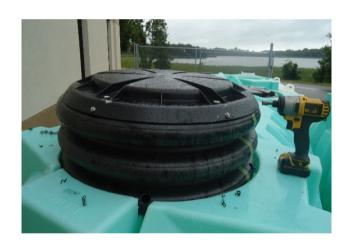
12. For a water tight lid seal, apply foam tape on the underside of lid prior to attaching lid to pipe.
