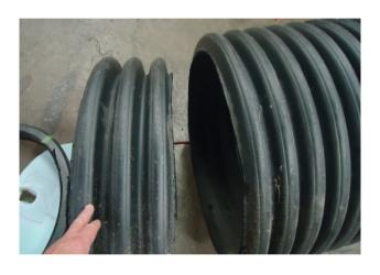
3. Insert pipe on tank manway, ensure it is centered and completely seated.
