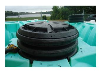
10. Caulk holes shut at 6 locations where original lid screws were used. Using original lid screws, fasten lid to pipe in locations as shown.
