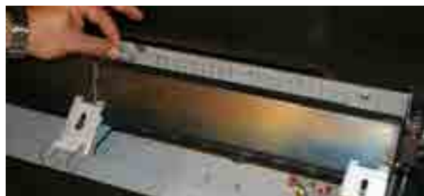
Figure 22. Closed Vane for Top Vent Fireplaces.
