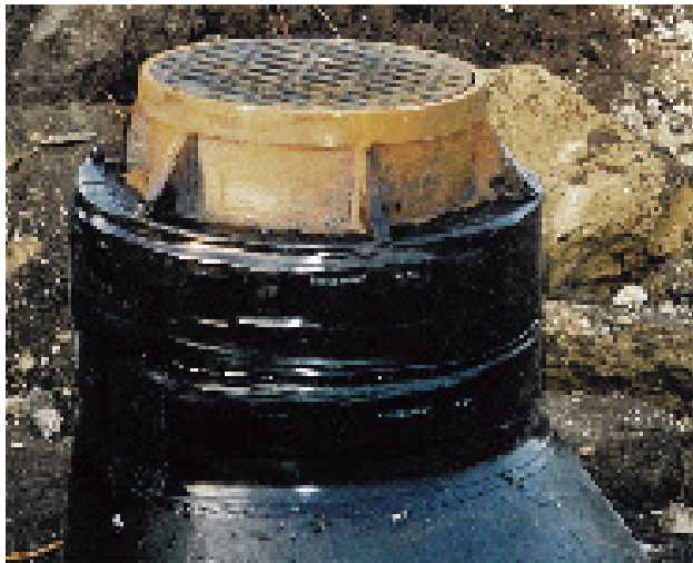
High shrink membrane conforms to irregular structures.
