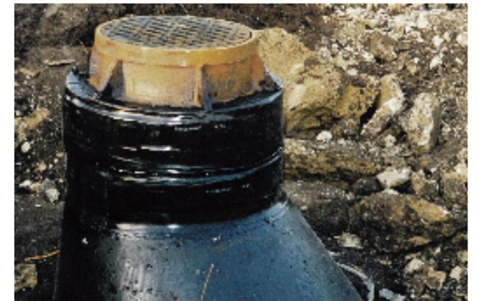
*WrapidSeal™ reduces I & I and provides long term manhole integrity.*
