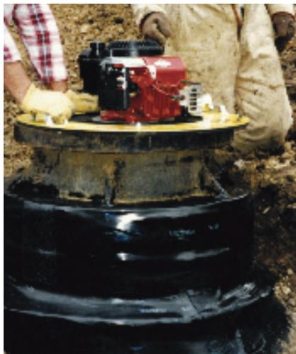
*WrapidSeal™ - positive external seal; vacuum tests to 11" Hg.*
