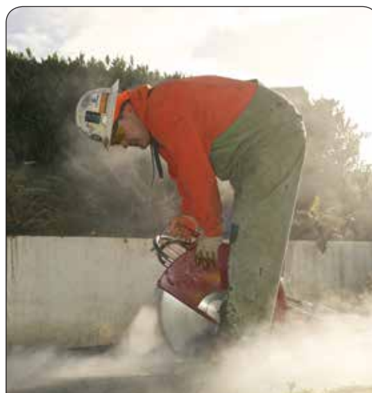
Hand sawing with a Wolverine hydraulic handsaw
