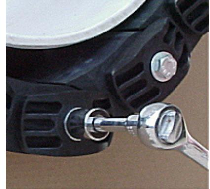
1. Center the pipe, cable or conduit in wall sleeve, casing or core drilled hole. Make sure the pipe will be adequately supported on both ends. Innerlynx are not intended to support the weight of the pipe.
