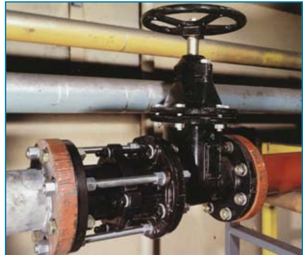
4" Dismantling Joint in plant room application
