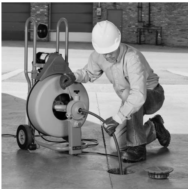
Figure 14 – Operating the K-750 using the AUTOFEED
