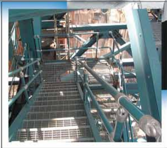
For OSHA regulated areas, Speed-Rail® is the most frequently used product, often in conjunction with galvanized steel pipe.
